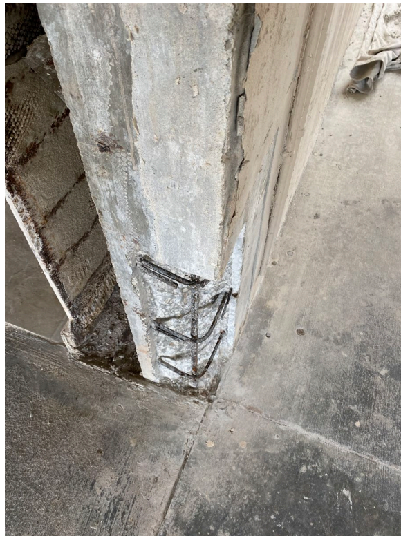
Picture 2: Typical wall repair
