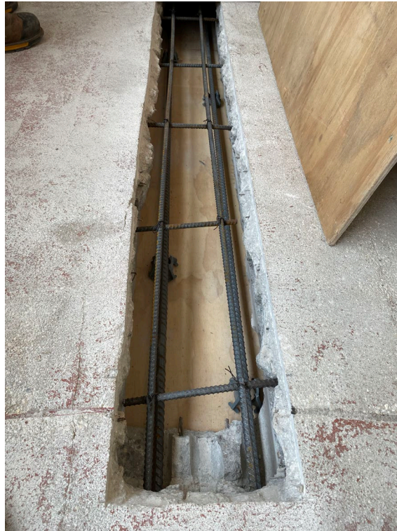
Picture 3: Full depth 1 st floor walkway repair
